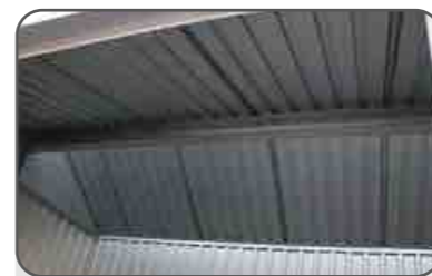
Strong Steel Roof Truss Carries 18 lbs /sq.ft. Snow Load
