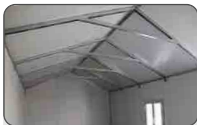
Strong Steel Roof Truss Carries 30 lb/sq.ft. Snow Load
