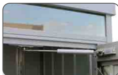
Hydraulic Gas Cylinders to Keep Doors Open
