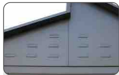
Built-in Dual Slotted Air Ventilation System
